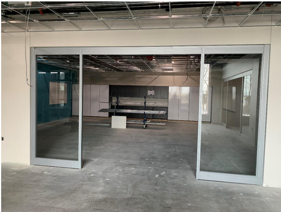
12. Area 4 – Sliding door system install in second floor classrooms in progress.
