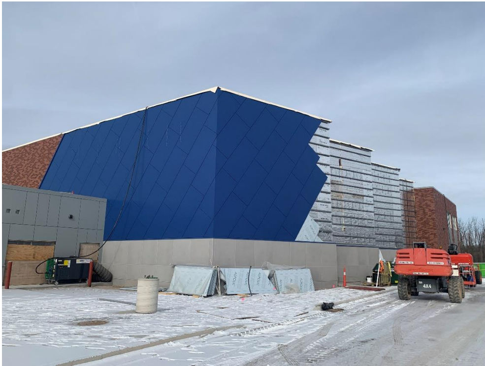
2. Area 2B – Composite wall panel install on upper soffit at Fitness Room continues.
