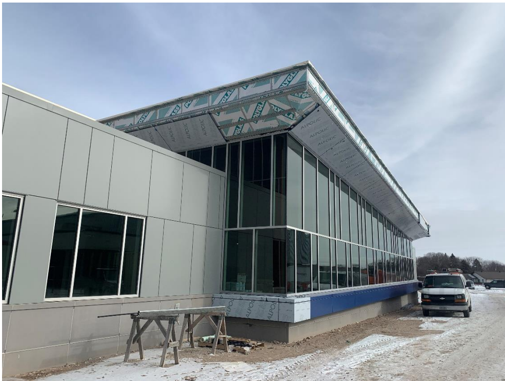
2. Area 2B – Composite wall panel install on upper soffit at Fitness Room continues.
