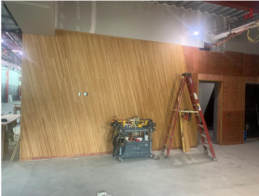
5. Area 1A – Wood plank install in center spine in progress.
