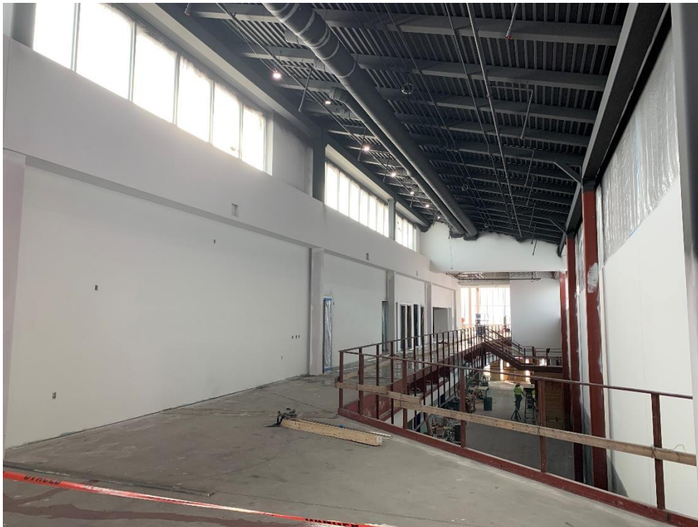
6. Area 1A/1B – Painting in center spine in progress. Terrazzo flooring install is beginning.
