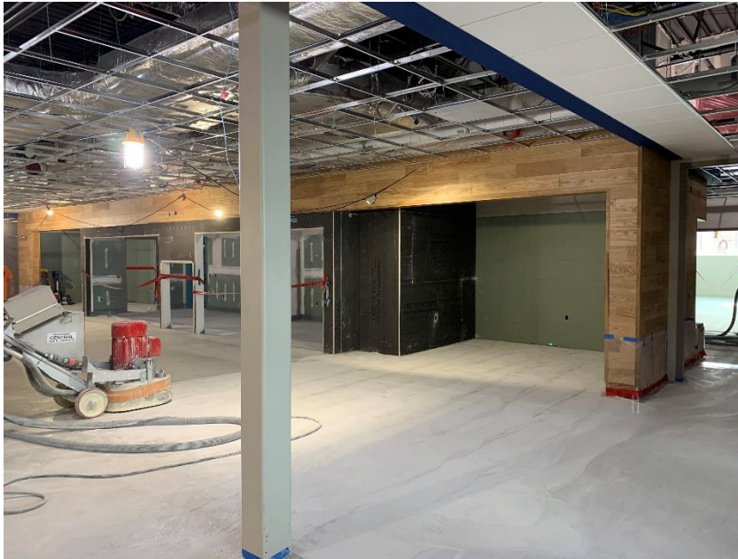
9. Area 4 – Painting and terrazzo flooring install in the second floor flex café in progress.
