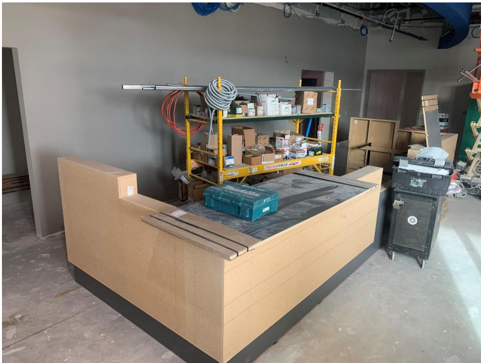
4. Area 1A – Casework and reception desk install in progress.
